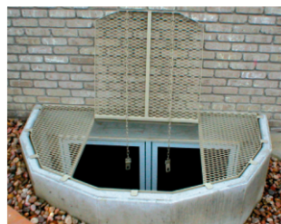
EMERGENCY EGRESS ESCAPE HATCH
